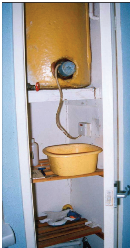
Airing cupboard with hot water tank above
